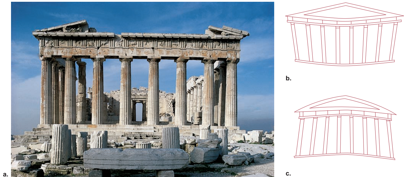
FIGURE 5 In building the Parthenon, the Greeks constructed an architectural wonder that looks perfectly straight, with right angles at every corner, as in (a). However, if it had been built with completely true right angles, it would have looked as it does in (b). To compensate for this illusion, the Parthenon was designed to have a slight upward curvature, as shown in (c). (Source: Coren & Ward, 1989, p. 5.)
