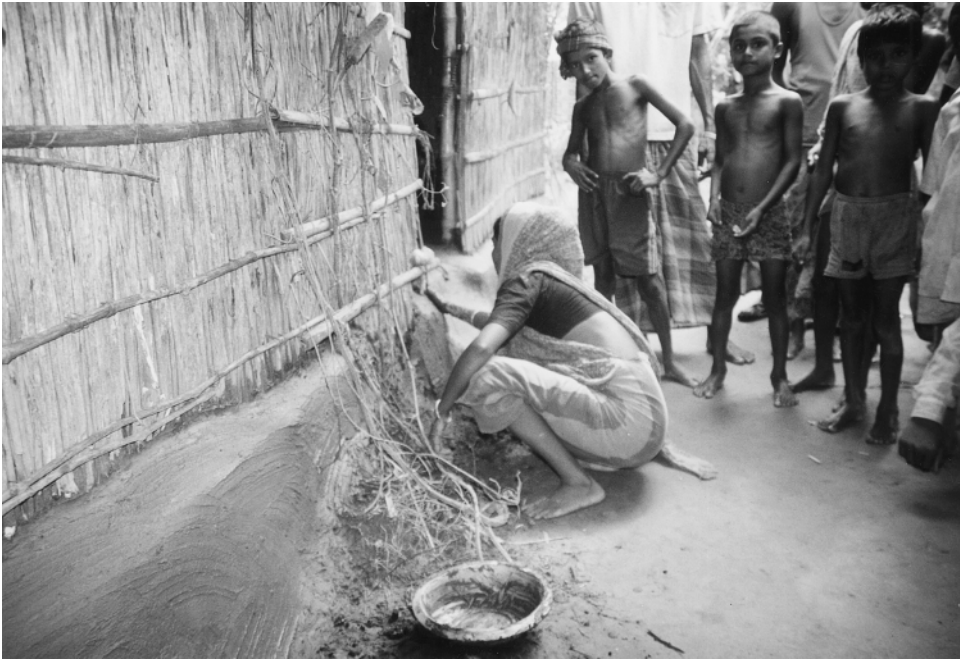
Plate 5.5 Bangladesh: a woman applying a new layer of mud to strengthen the foundation of her house during the monsoon season, when flooding is common. Her husband is a handloom weaver as the family has no land, so the wife is responsible for all outdoor work as well as housework and childcare.
