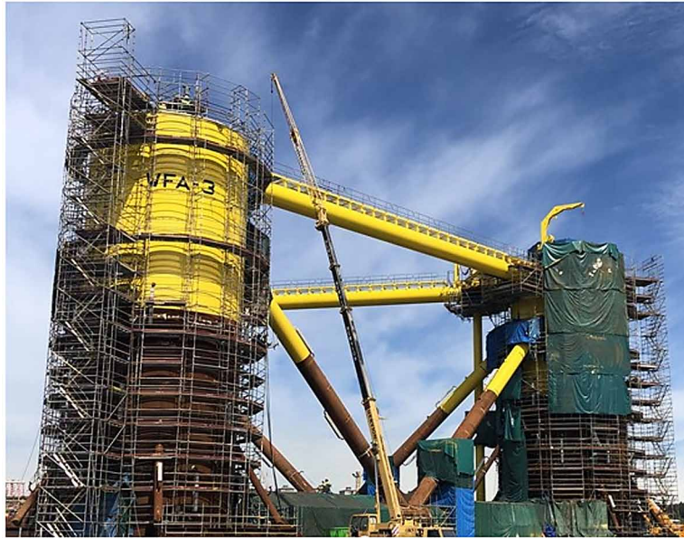
Figure 1. Building the floating offshore wind platform called WindFloat for the WindFloat Atlantic project in a shipyard.
